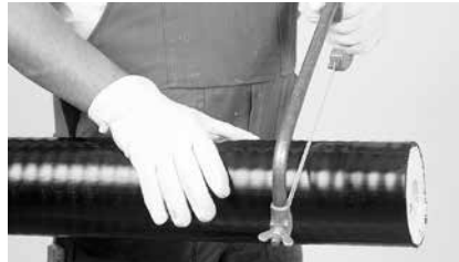
2 Cut the casing pipe with saw.
